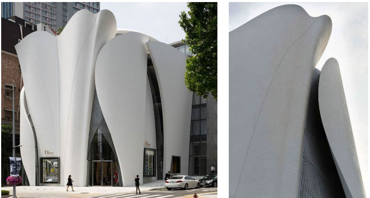
Figure 1.1. Example of Fiberglass fabricated panel structure: The House of Dior in Seoul, South
